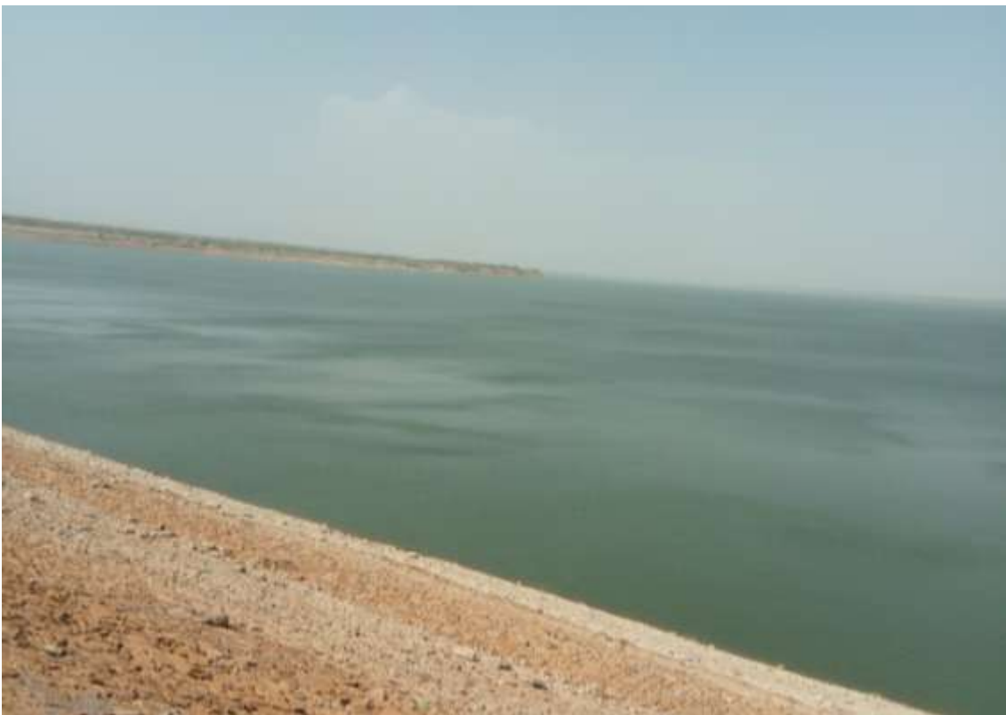
Fig. 6. A view of Hub Dam.
